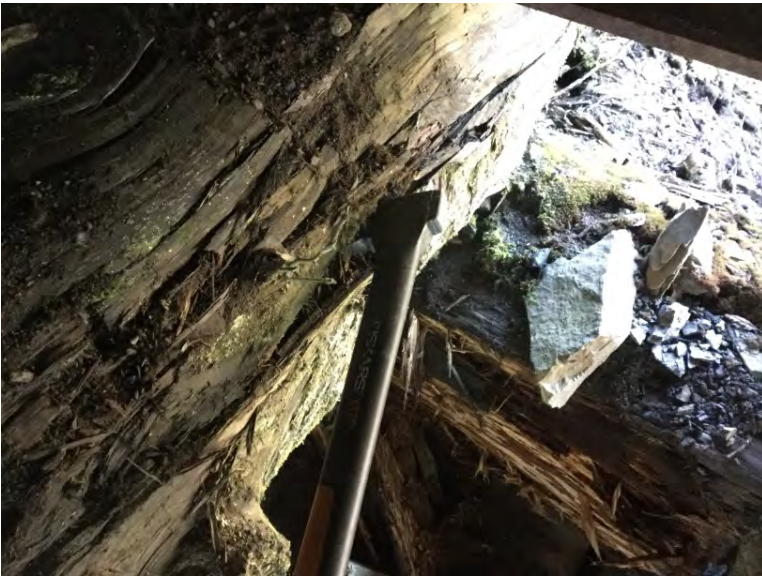
Up to 70mm sap rot in face logs and tiebacks
