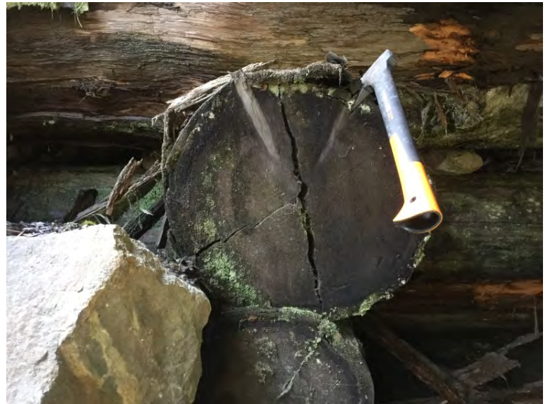
Tieback ends spilt and up to 70mm sap rot
