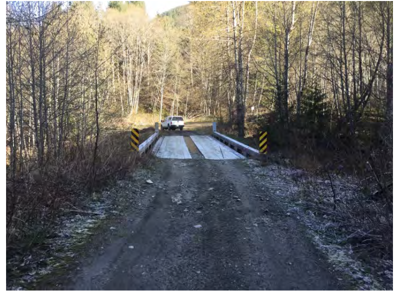
Approach from Left Bank when facing downstream
