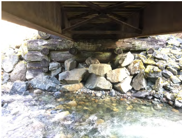
Right Bank Abutment when facing downstream
